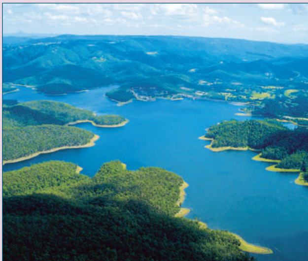
figure wq.2 The Hinze Dam supplies water to the Gold Coast. It has a catchment area of 207 km 2 , a storage capacity of 163 500 million litres and a surface area of 972 hectares. It was originally built in 1976 and the wall was raised a further 18 metres in 1989.
