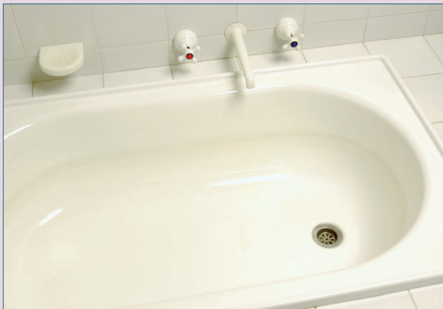
figure wq.6 Hard water is generally a result of the geology of the local area rather than pollutants. Magnesium and calcium ions in water react with soaps and detergents producing the scum that forms in a bath or shower. They also mean that greater amounts of detergents are needed to wash clothes. The build up of magnesium and calcium compounds as scale in water pipes can also cause problems for local councils.
